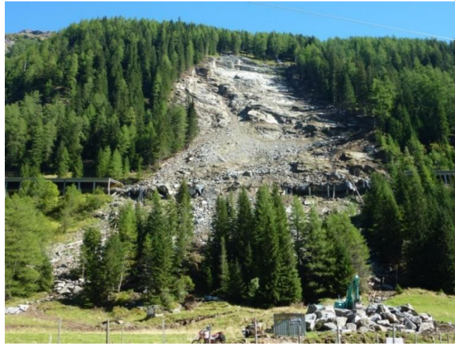
Fig. 2: The Felbertauern rockslide with destroyed road and gallery, photo from September 2013
